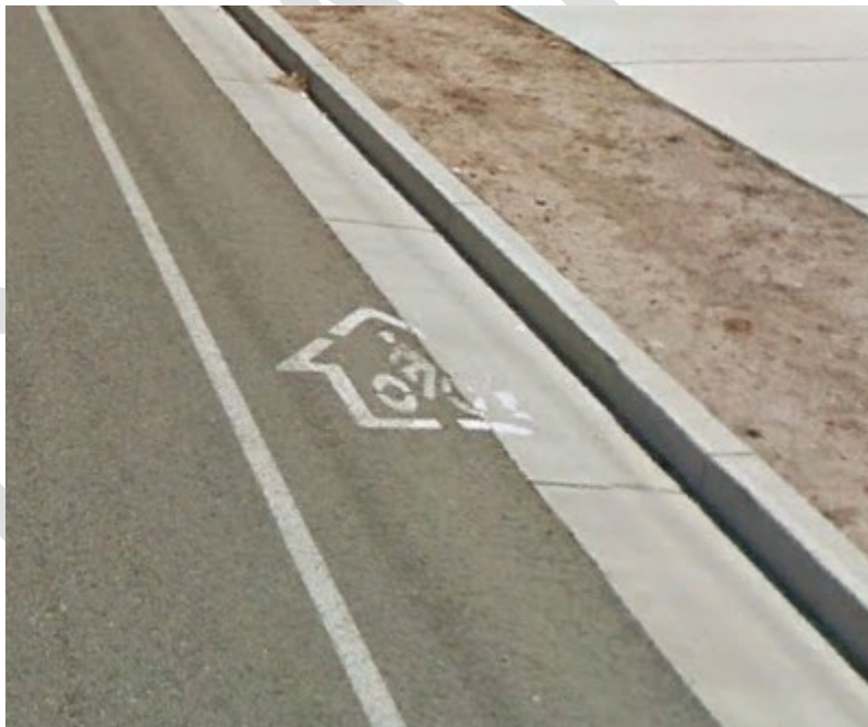
Figure 3.17: Striped Shoulder Bike Lane in Moab
